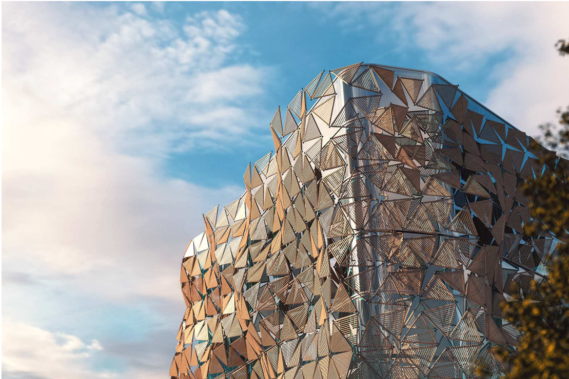
Figure 3.18 – A free-form facade constructed from uniform triangular elements connected with rotational joints. Thanks to the reconfigurable nature of the regular auxetic linkage, the facade can be used as a computer-controlled dynamic external shading system.
