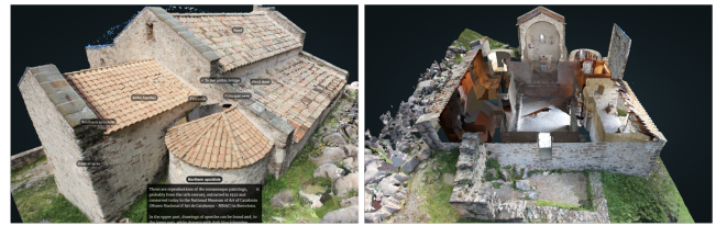
Figure 9: Inspection of St Quirze de Pedret pointcloud.
