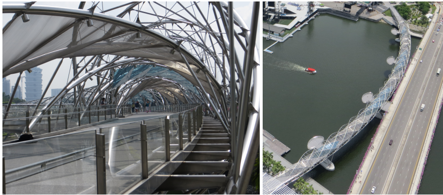
Figure 2.4: The Helix Bridge is a pedestrian bridge in the Marina Bay area in Singapore. Its generative design has been optimized numerically. Furthermore, the bridge was fully modeled in order to visualize its form and geometric compatibility, as well as to visualize the pedestrian experience on the bridge. Photo kindly provided by Volker Settgast.
