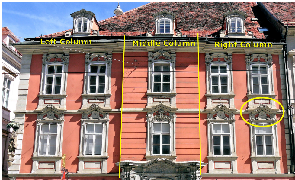
Figure 1.1: An example of a façade in the city of Graz, Austria. We can observe several symmetries in the architectural design: similar windows with different ornaments above – see also the encircled example – a middle column with symmetric parts left and right, and similarly structured elements like columns and ornaments (photo by author).
