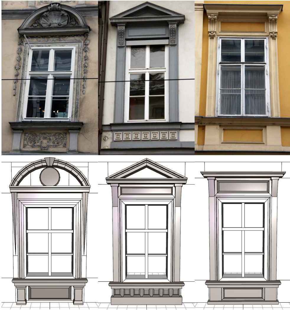
Figure 5.2: Different window styles using the shape grammar system based on convex polyhedra (modeled by Rene Zmugg).
