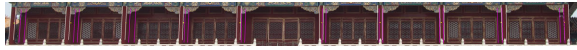
Figure 6: Column segmentation. The yellow points are the initial locations of outer columns. After refinement, the final inner columns and outer columns are marked by magenta lines and white line respectively.
