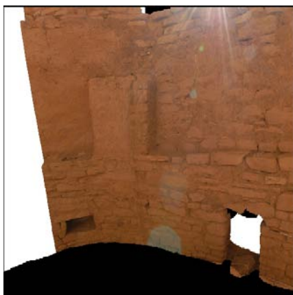
Figure 6: The result of texture mapping the kiva scan with the photograph in Figure 1b. The mapping aligned well with the extruded pillar like structures on the kiva wall as well as the border between the kiva wall and the floor.
