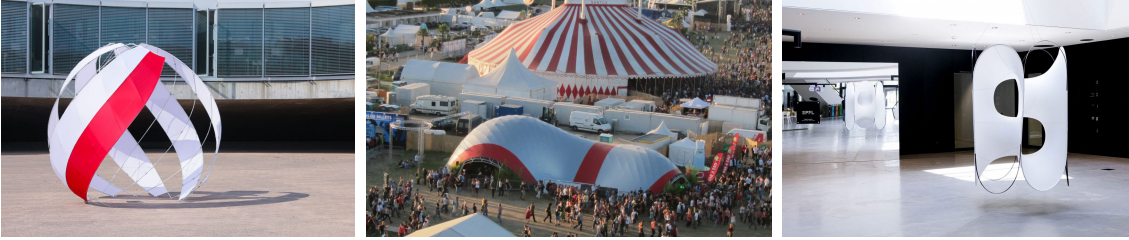
Figure 6.2: Example of elastic structures combined with surface elements. From left to right: The X-shell pavilion by Isvoranu and colleagues 2019, the Solidays Forum by the THINKSHELL group [Baverel et al., 2012], and the el.ba by Alison Martin and the EPFL Geometric Computing Laboratory.
