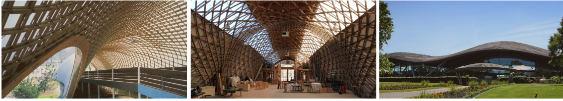
Figure 1.2: Examples of three large-scale gridshells. From left to right: The Multihalle in Mannheim, the Weald and Downland Gridshell Building in Singleton, and the Savill Building in Windsor. Photo credits can be found in Appendix C.
