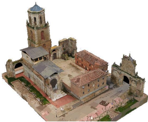
Figure 6: 3D model of the current state of the monastery remains. This model results from merging terrestrial and aerial photogrammetry with laser scan data.
