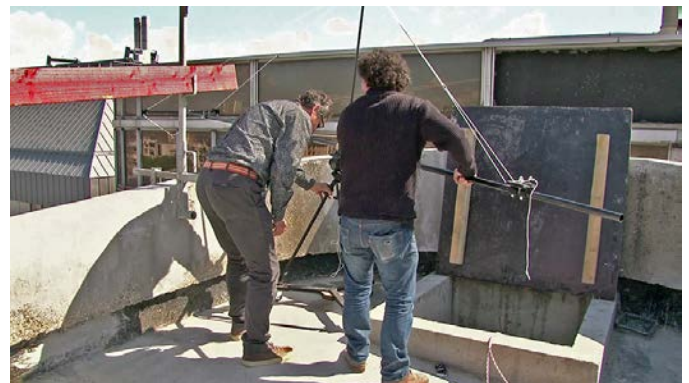
Fig. 3. Installing the crane on the roof-top
