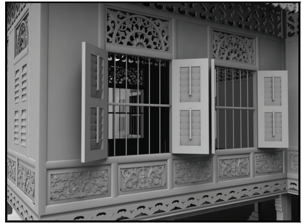
Fig. 16 Another beautiful carving found in Rumah Tok Su, combination of kerawang tebuk and kerawang timbul.
