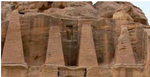
Figure 4: Statue and back face of the Obelisk facade. Water down flow on the surface, alveolar weathering on the right, with weathering granular disintegration and loss of form at statue
