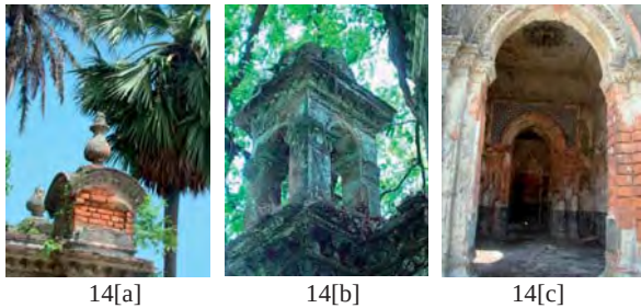
Figure 14: [a] Bengali Chowchala dome [b] Kiosks [c] Entry of Larger Temple
