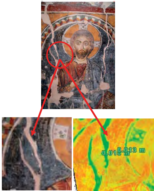
Figure 15: Monitoring the crack of the background of the fresco at Saint Kirikos and Ioulitis through Laser Scanners
