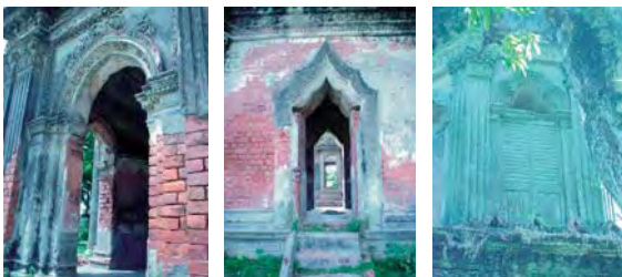
Figure 15(a): View of different types of Arches
