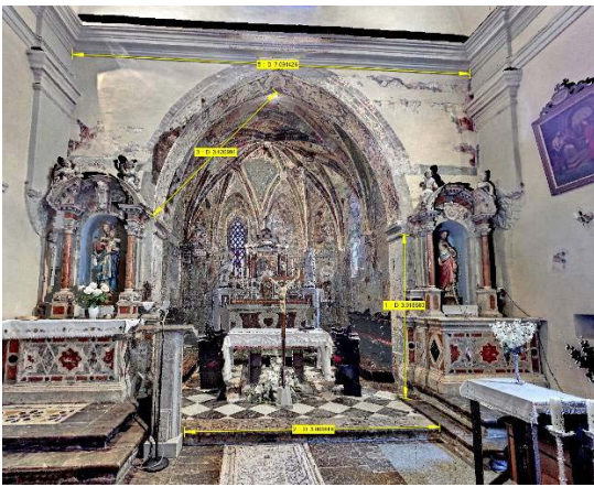
Fig. 2. 3D colored point cloud of the church interior
