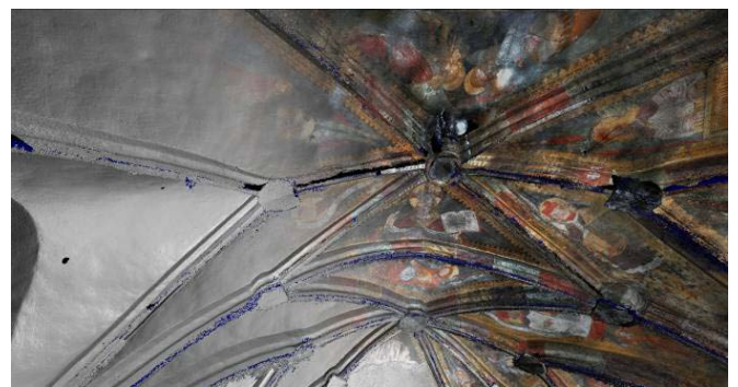
Fig. 4. 3D polygonal model of the vault with textures
