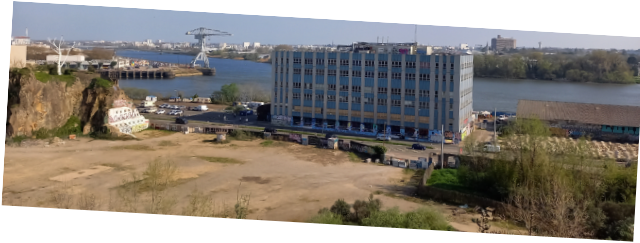
Figure 3: CAP44 before rehabilitation
