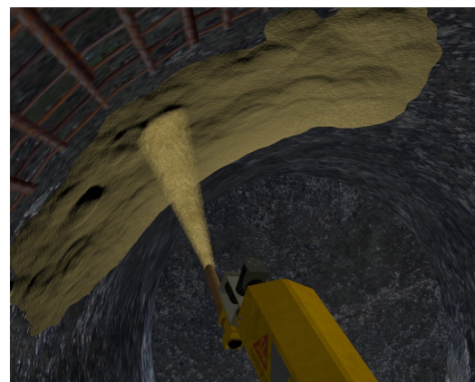
Figure 11: Sprayed tunnel wall.
