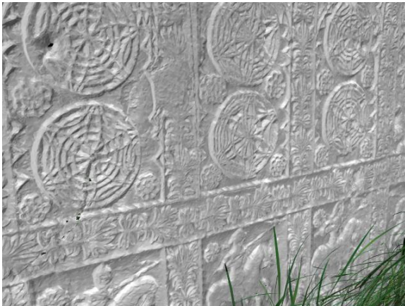
Figure 9. Incorrect orientation, 12:00 –close up
