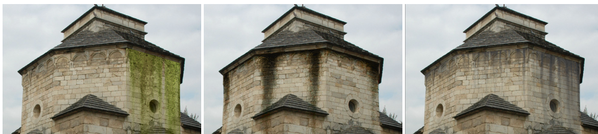
Figure 8: Chapel example: different applications of flow stains on a chapel image, including a biological stain and two moisture stains.
