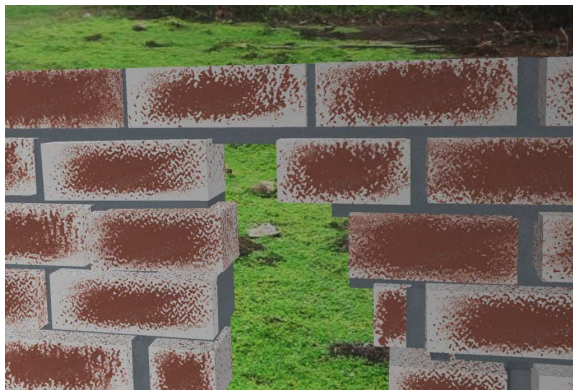
Figure 10: An old wall, affected with efflorescence. We have also applied this weathering process to mortar.
