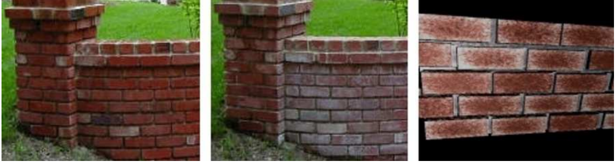
Figure 5: A real brick wall. On the left a clean version and on the middle, the same wall attacked by efflorescence. On the right: a wall synthesized by our method.
