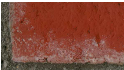
Figure 3: Zoom on a real fired-clay brick attacked by efflorescence: bump mapping is sufficient to handle these specific efflorescence geometric variations.
