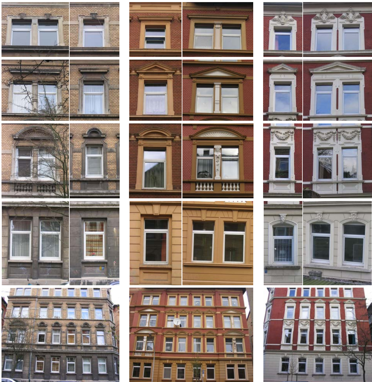
Figure 1.5: Structural similarity. Despite their diversity all Wilmerding buildings share some essential properties.
