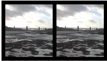
(g) Menai bridge
