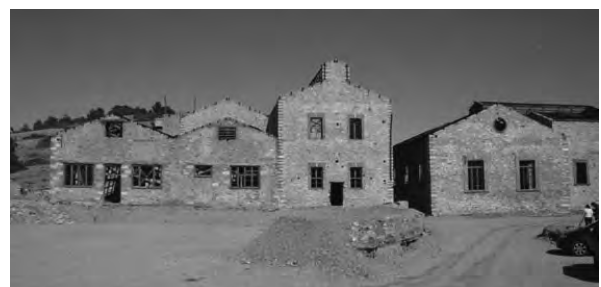
Figure 4: The buildings in the Technological and Cultural Park of NTUA in Lavrio
