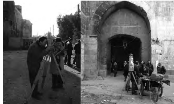
Figure 2: Laser scanning of the wall in vertical position and capture of the target coordinates
